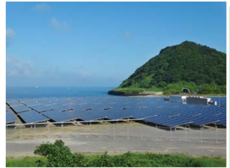
SoftBank Nagasaki Koyagi Solar Park
